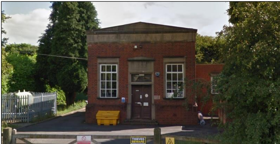
Figure 14: Locally Listed Pumping Station
