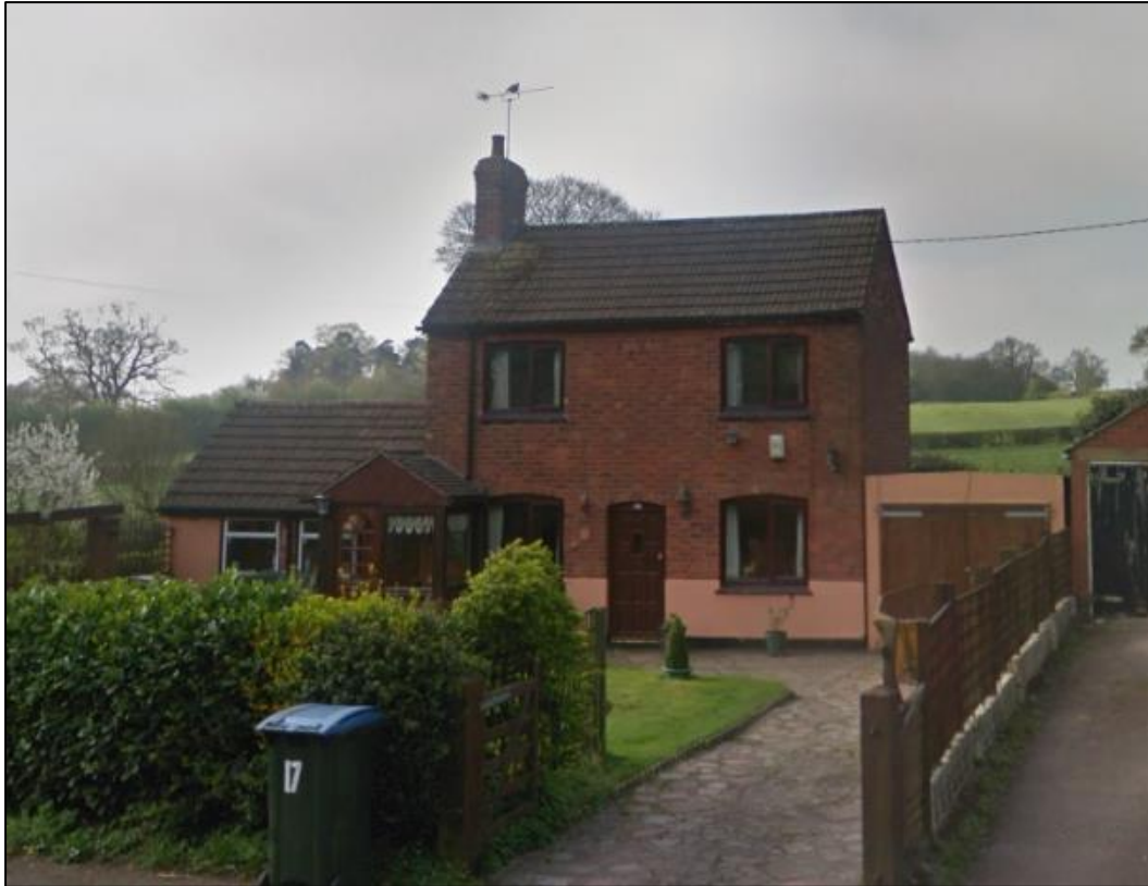
Figure 7: 17 Wall Hill Road
