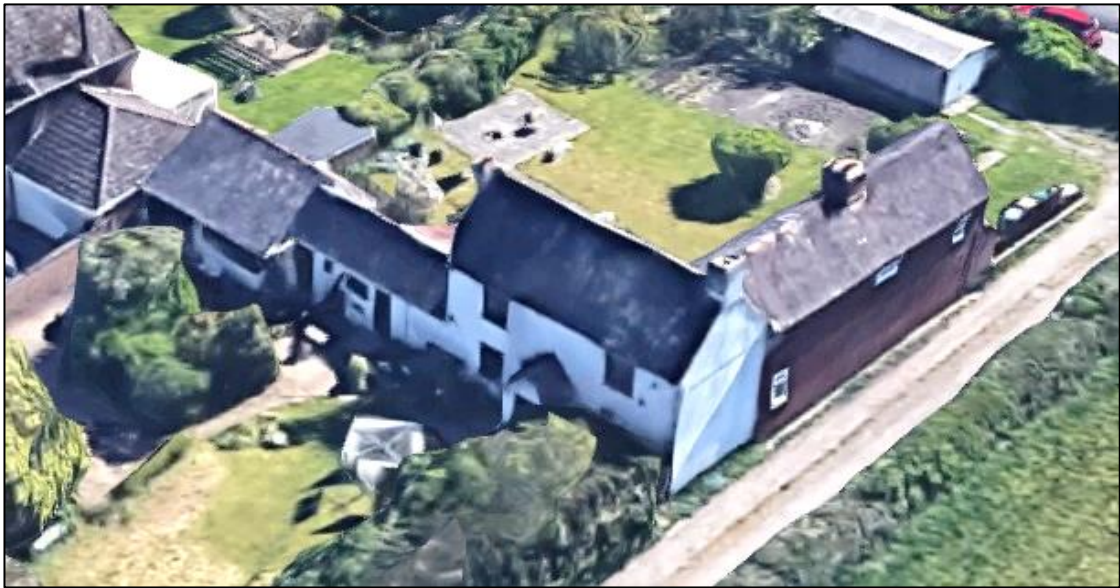
Figure 9: 29, 31 & 33 Wall Hill Road
